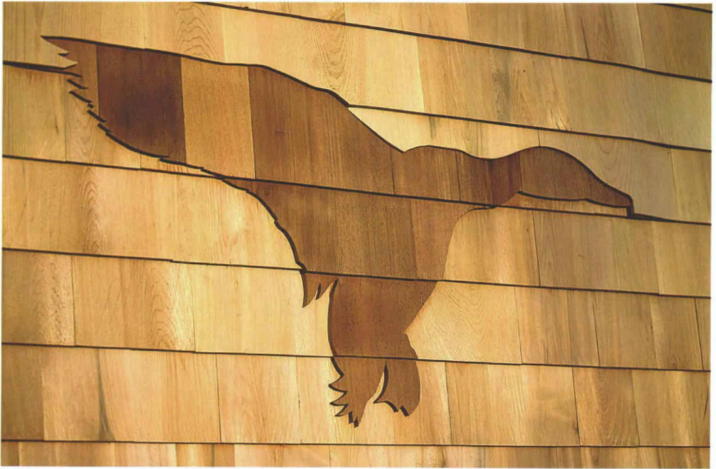
A strong silhouette makes a pleasing image. Images between 8 sq. ft. and 20 sq. ft. such as this duck work best for shingle designs. Red-cedar duck shingles overlap the white-cedar courses below to create the duck in relief.
