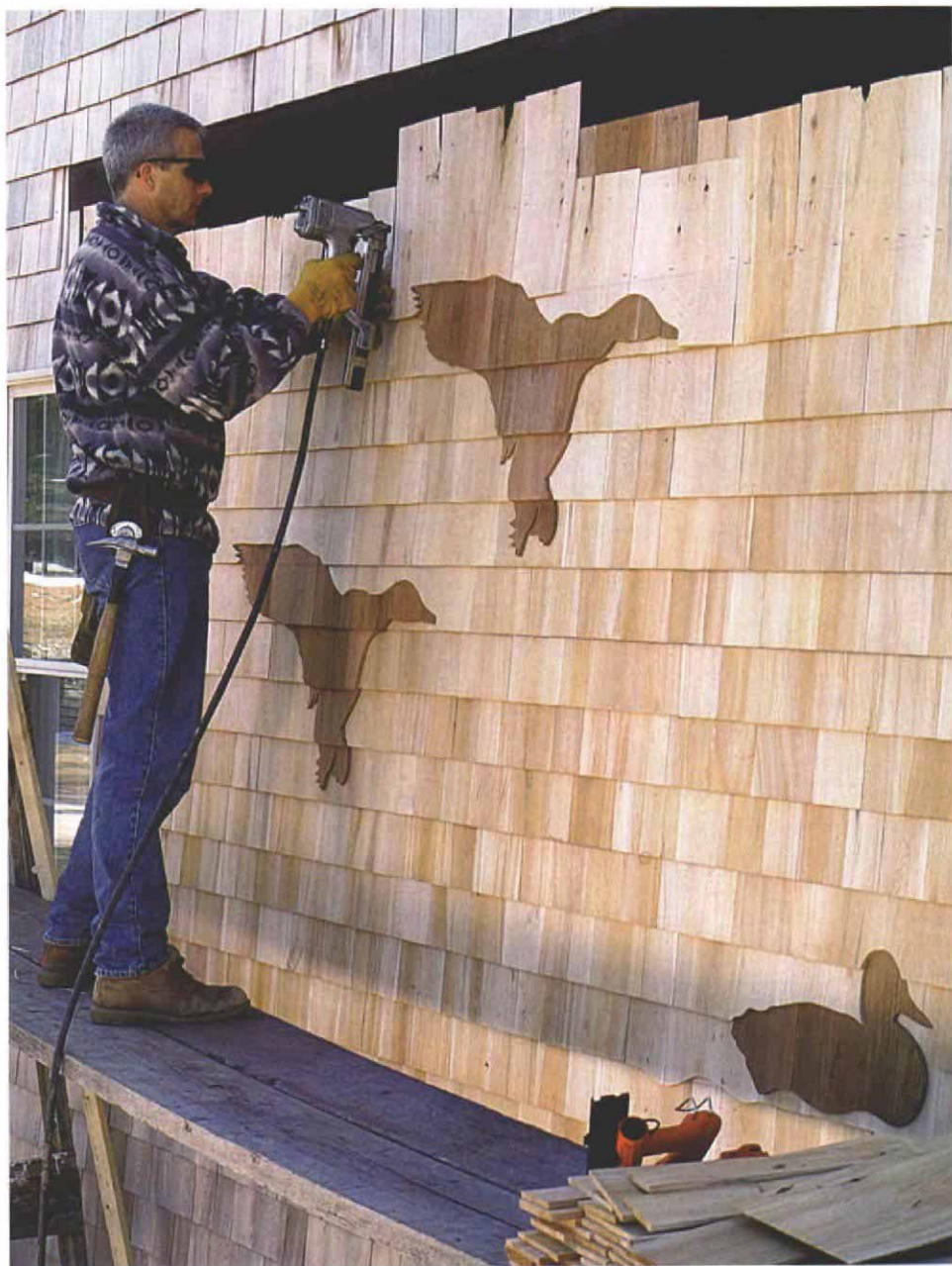
Nailing ducks in flight. Red-cedar shingles against a white-cedar background as well as various shingling techniques effectively outline the images of the ducks.
